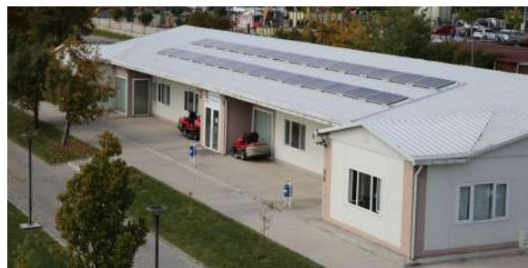
The Solar Power Plant Built on the Department Building's Roof
