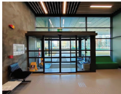
Tactile surface application
